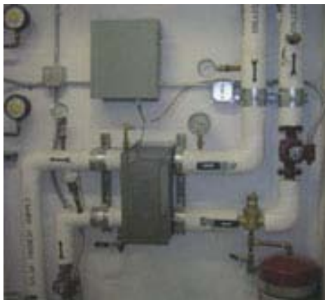
Photo: Solar plate heat exchange, Geo H. Wilson, Inc., http://www.geohwilson.com
